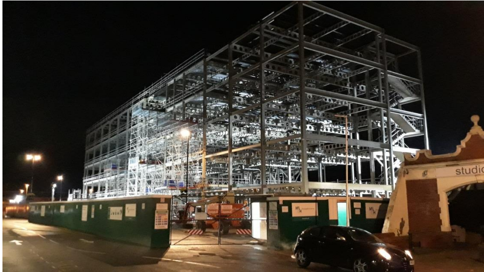
Teville Gate House Construction 12/12/2019
